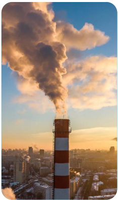
Post-combustion capture (PCC)
